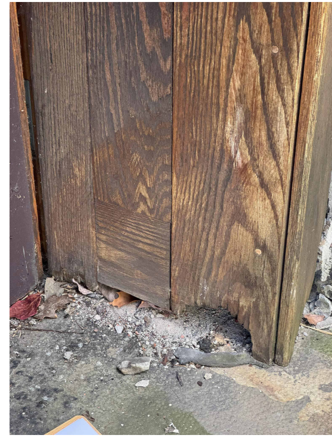
05 EXISTING NORTH EXTERIOR DOOR CASING, WEST SIDE, BASE 1 1/2" = 1'-0"
