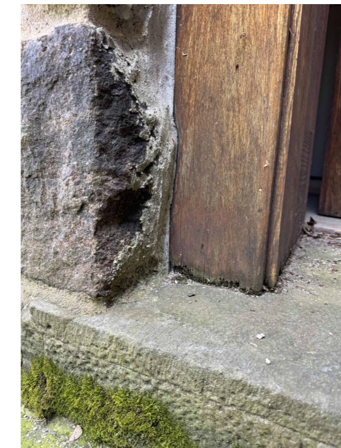
02 EXISTING NORTH EXTERIOR DOOR CASING, EAST SIDE, BASE 1 1/2" = 1'-0"
