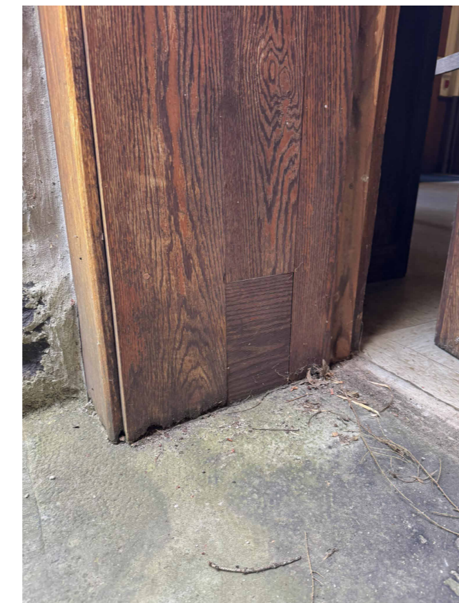
03 EXISTING NORTH EXTERIOR DOOR CASING, EAST SIDE, BASE 2 1 1/2" = 1'-0"
