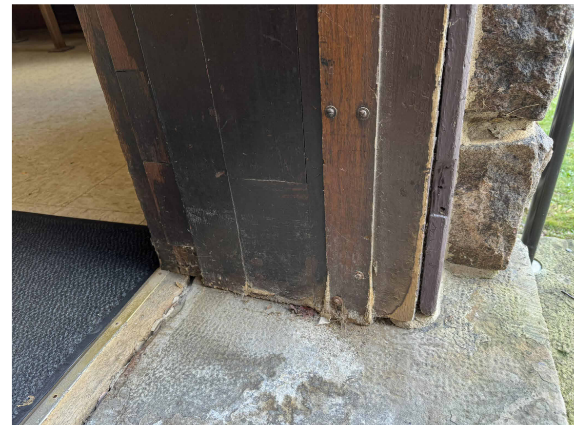
11 EXISTING EAST EXTERIOR DOOR CASING, NORTH SIDE, BASE 1 1/2" = 1'-0"
